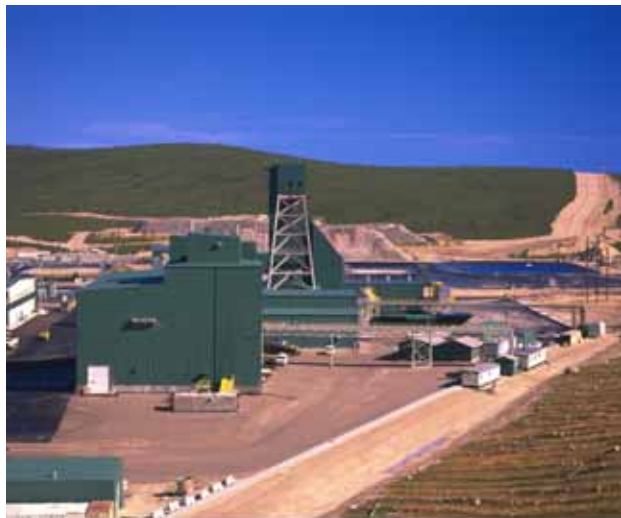
McArthur River McArthur River is the world's largest, high-grade uranium deposit. The headframe in the photo is over the #1, or Pollock shaft, which is used to access underground tunnels at the 530 metre level and the 640 metre level.
