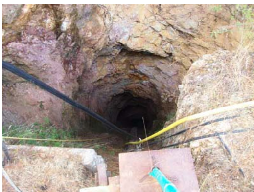
Figure 7—Historic San Luis Mine Shaft, Current Water Supply for Town of Guazapares Source: Analyst
